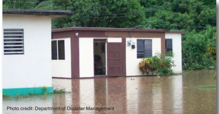
Photo credit: Department of Disaster Management
